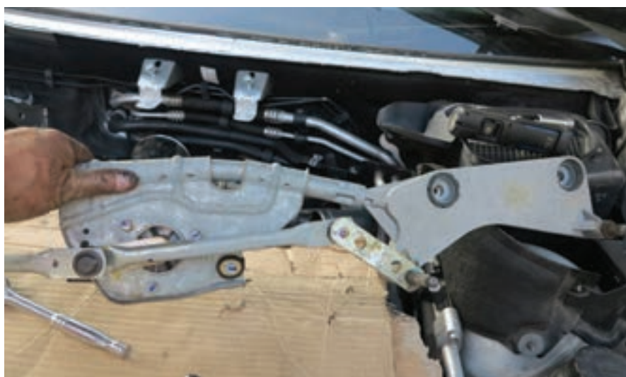
2. Removing the wiper mechanism.
